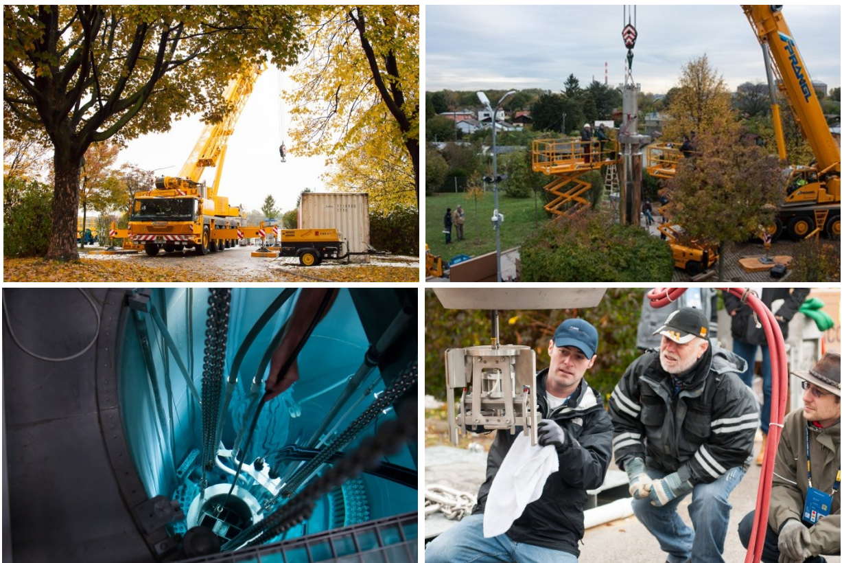
1.1 Exchange of the fuel elements
